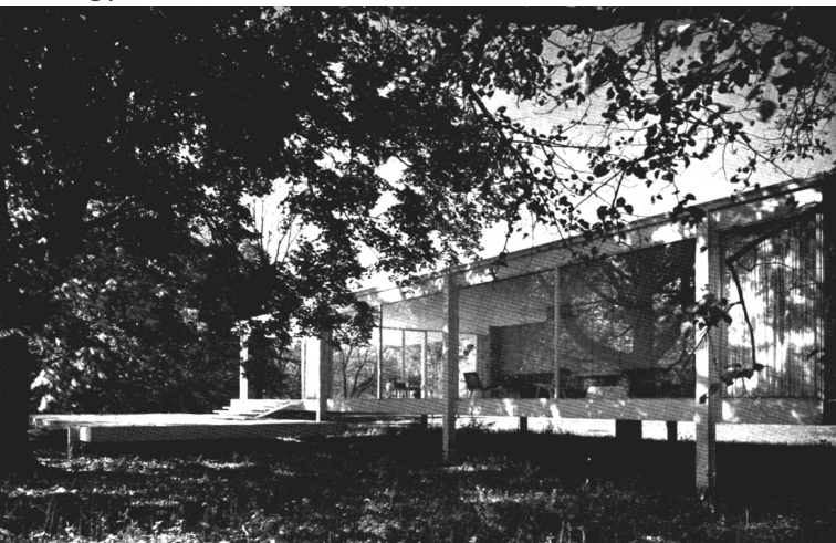
What Mies was best at: glass boxes and bubbles in primordial, dehumanised space. Somewhere to 'get away' from the Architecturally illiterate lifestace-design culture of 'stack 'em high and sell 'em cheap' - like over to the Right...
