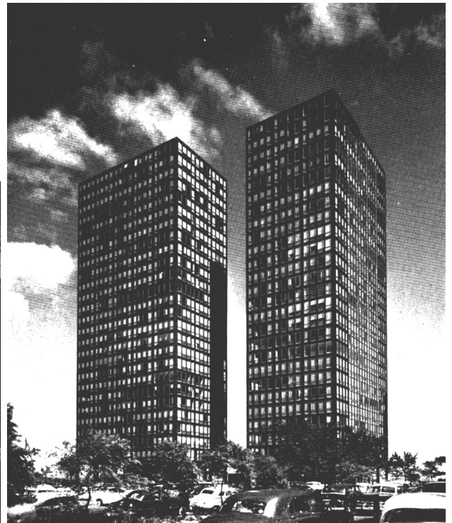
Domestic silo-stacks. The view down is of the Garden of Ballistics: Corbusian Espace, Verdure, Soleil et automobile parking, freeways and bits and bobs of inaccessible 'Parkland' vegetation.
